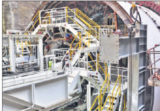
Weighing around 3,100 tonnes and measuring 96 metres in length, the machine is among the largest ever deployed for a railway tunnelling project in India.
