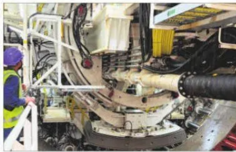
A tunnel boring machine being used for excavation.
